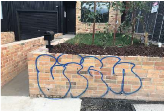
New wall protected with Nanoman Anti-Graffiti coating that has been freshly tagged.
