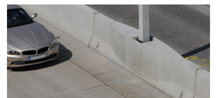
Light Mast Foundation
